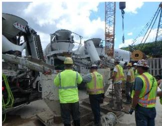
Concrete placement for cutoff wall panels.
