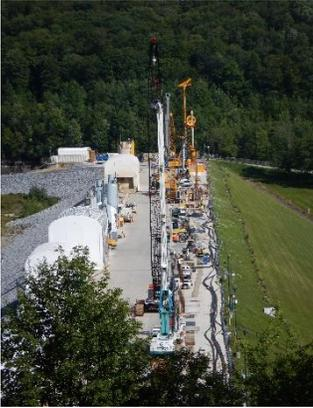
*Mix of drills and hydromill along left embankment.*
