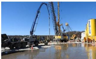
Concrete placement for secant piles using concrete boom pump truck.
